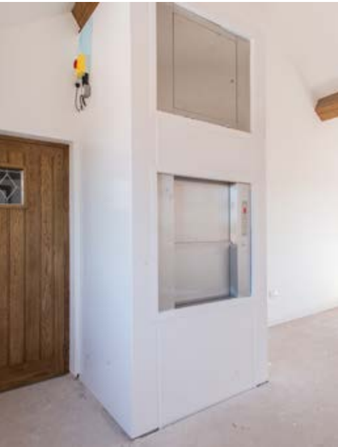
Self-contained dumbwaiter
